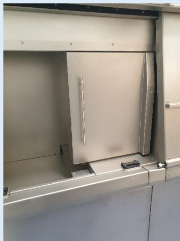
Position of Pass Through incl. 50mm lead door and status indicator for the alarm of the LAF in the sluice
