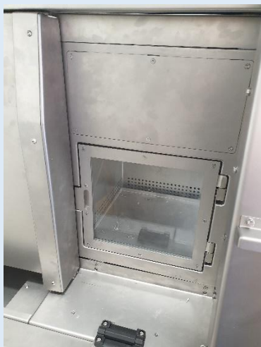
Position of Pass Through incl. 50mm lead door and status indicator for the alarm of the LAF in the sluice
