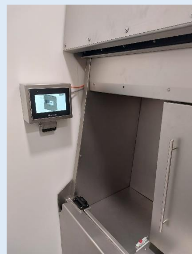
Position of Pass Through incl. 50mm lead door and status indicator for the alarm of the LAF in the sluice
